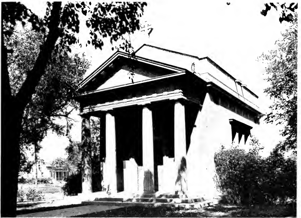
NEWELL MEMORIAL CHAPEL KENOSHA CEMETERY ASSOCIATION, KENOSHA, WIS. N. MAX DUNNING, ARCHITECT
